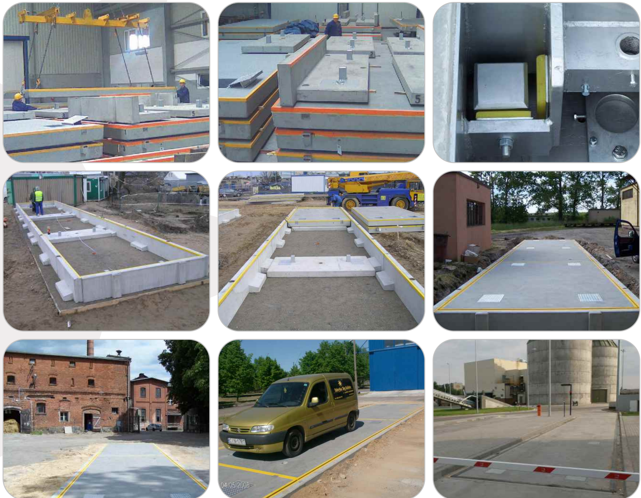
Assembly and installation phases of a concrete weighbridge
